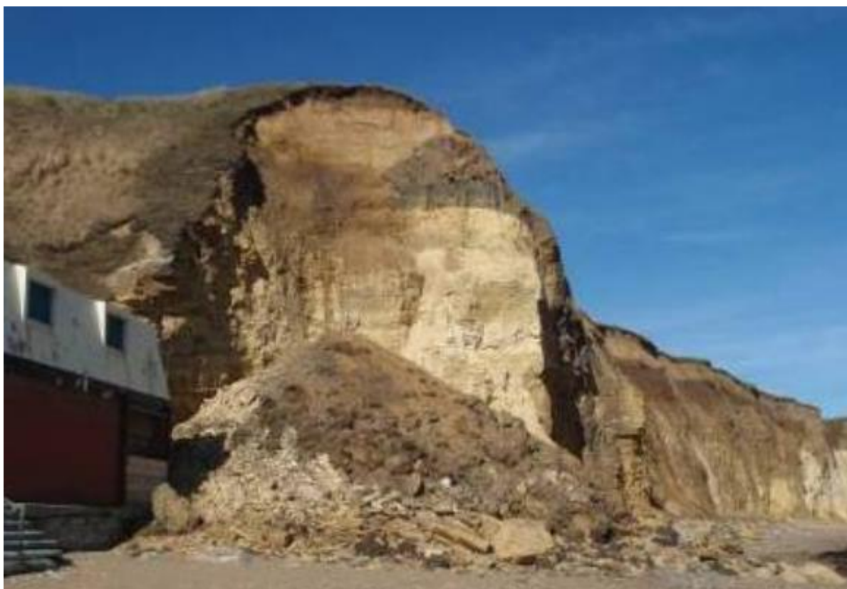
Figure 3-20 – Marsden Bay rockfall, 2010
