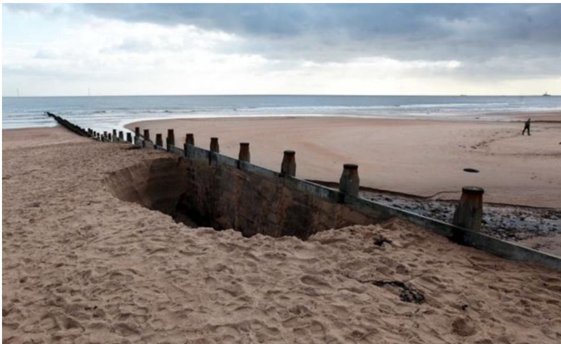
Figure 3-15 – Sink hole in the beach due to changes in the channel alignment of Meggies Burn, October 2019
