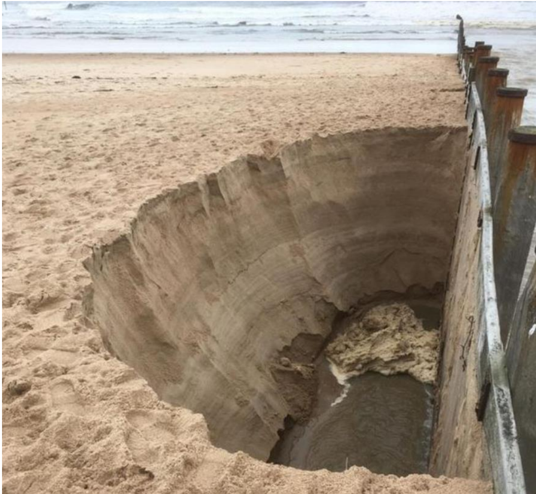
Figure 3-16 – Sink hole in the beach due to changes in the channel alignment of Meggies Burn, October 2019
