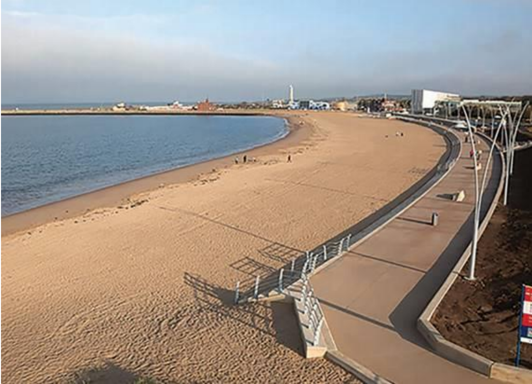
Littlehaven Promenade and Seawall, South Tyneside
