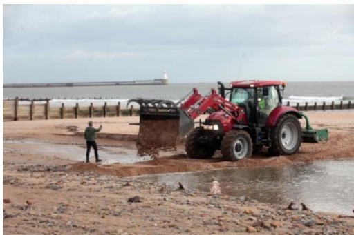
Figure 3-17 – Infilling of sink hole
